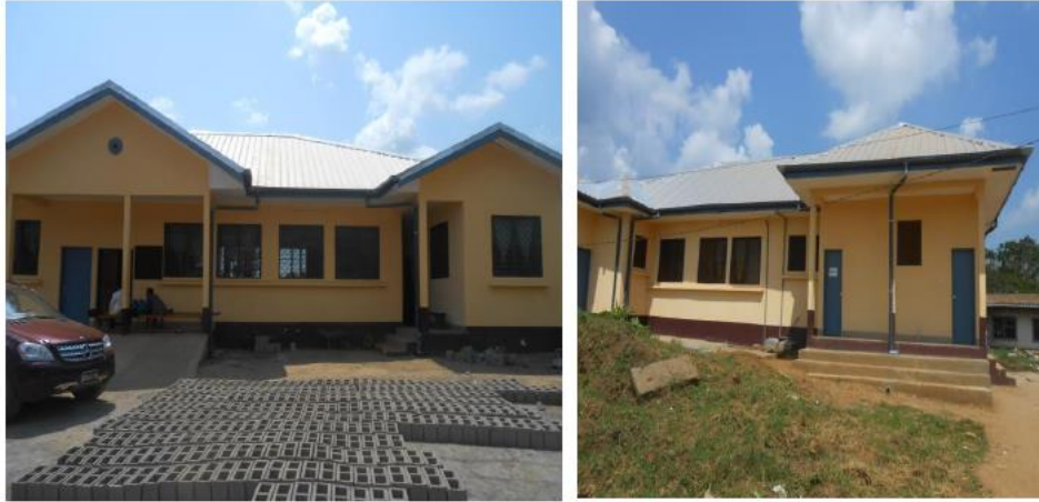
Figure 3. CMA after construction of the wards
